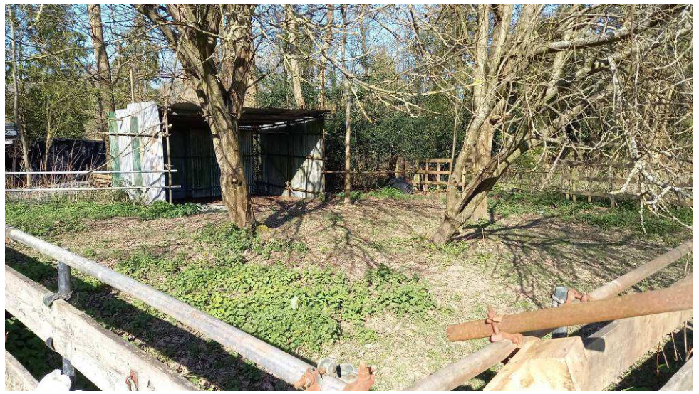
Photo 6 – Lean-to shed building in the NW
