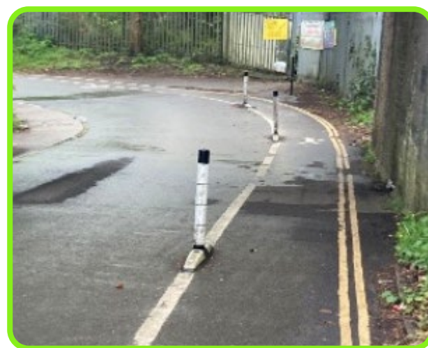
Figure 7-16: Implied footway protected by wands, Surrey.
