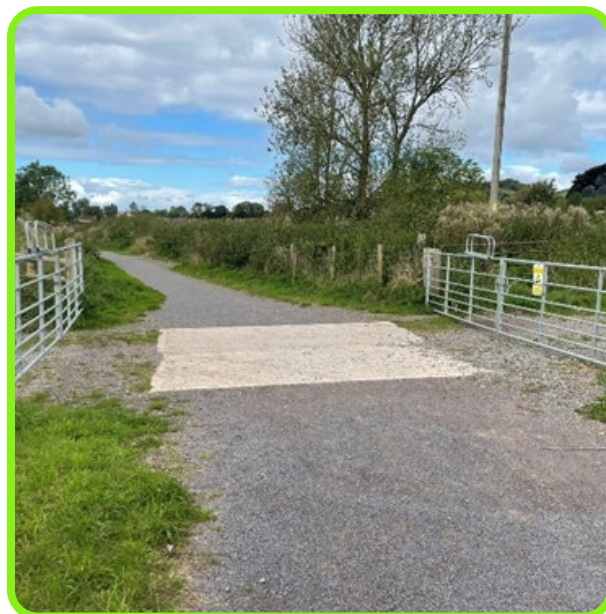
Figure 8-28: Concrete crossing pad and gates.
