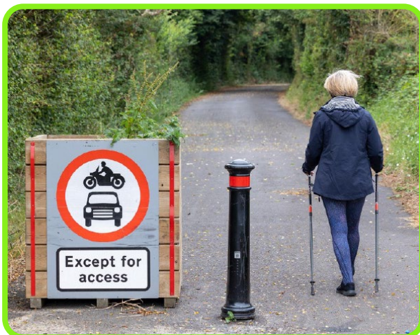
Figure 7-9: Rural modal filter introduced via an experimental traffic regulation order, Queen Charlton (Bath and North East Somerset).
