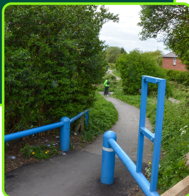
Figure 8-21: Shared-use path barriers in York.
