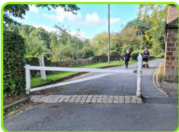
Figure 7-10: Traffic filter with gate for local access, Knaresborough.
