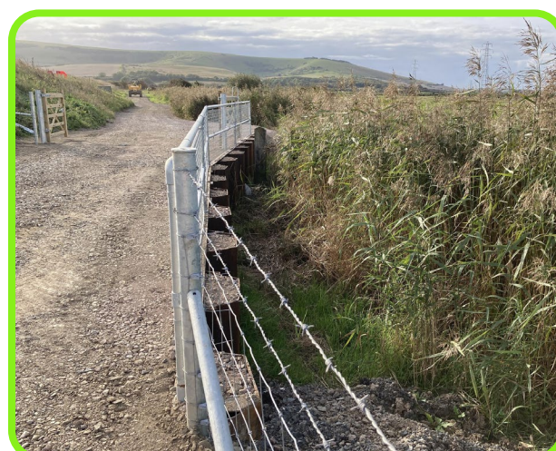
Figure 14-2: Sheet piling used to form part of route along Egret's Way, Sussex.
