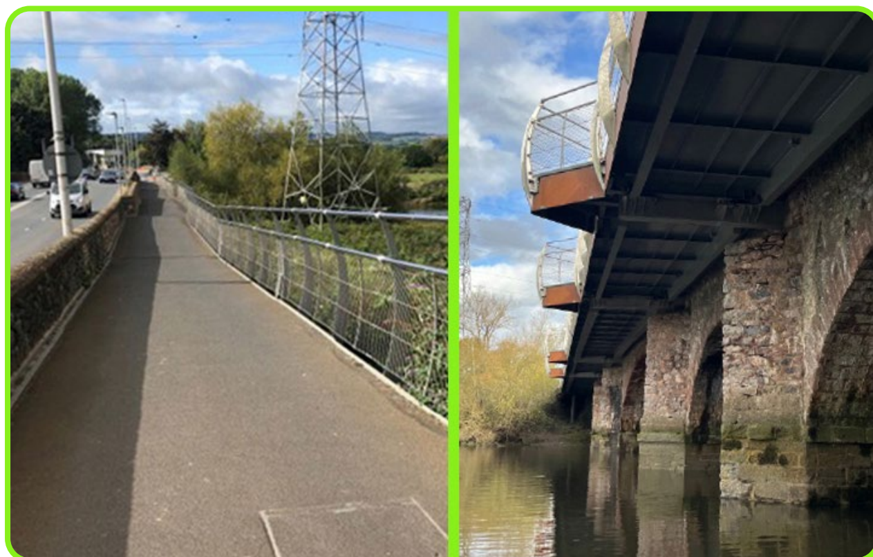
Figure 6-15: New active travel route cantilevered from the Countess Wear Bridge, Exeter.
