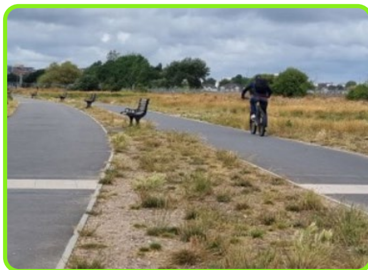
Figure 4-2: Separation by a vegetative barrier between cyclists (right) and pedestrians (left).
