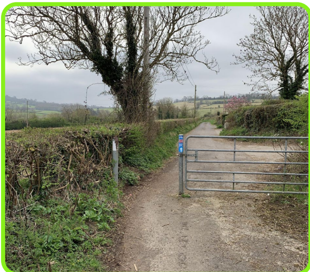
Figure 8-25: Gate and bollard arrangement – North Somerset.
