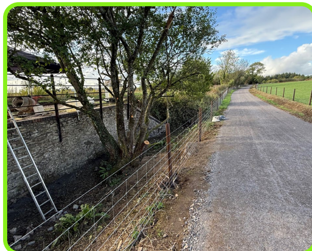
Figure 8-9: Shepton Mallet path running on field edge boundary where a farmer has retained the old rail bed for farm use on the left side of the fence.
