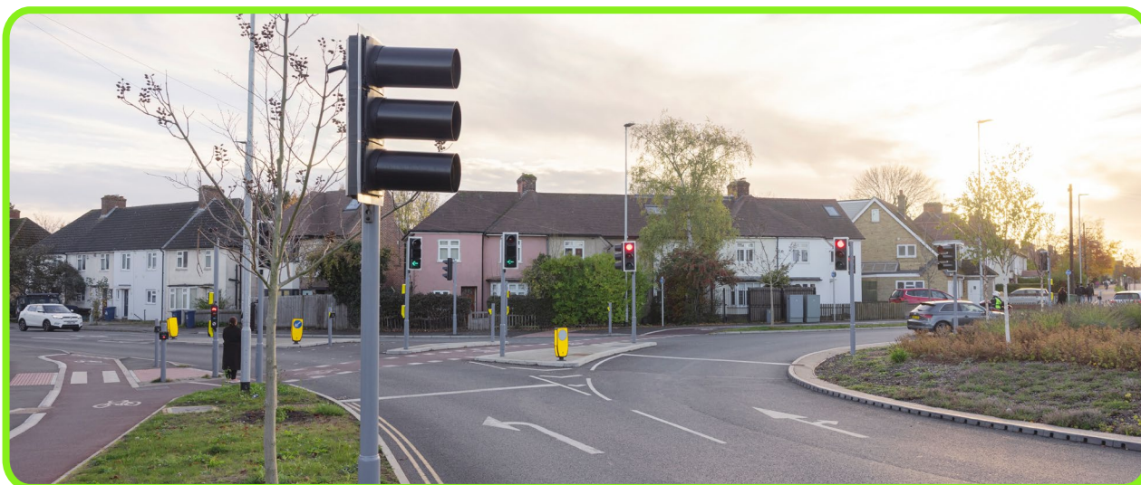
Figure 10-26: Roundabout with signal-controlled crossings, Cambridge.
