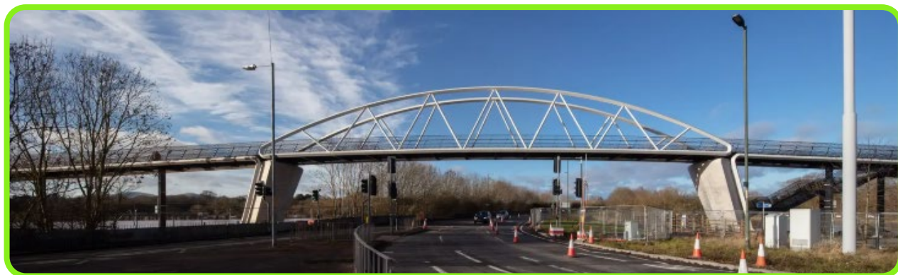
Figure 10-22: Hams Way bridge, Worcestershire.
